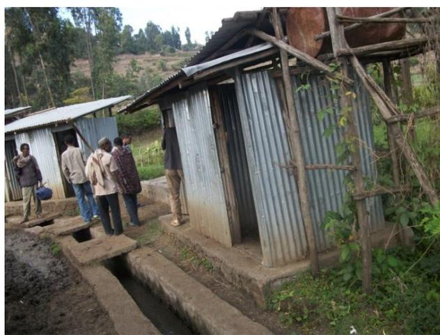
Poorly implemented gravity spring scheme provided with irrigation canal and shower at Tigo spring in Tehuledere *Woreda* (Photo by: Wondimu P., 2011)
