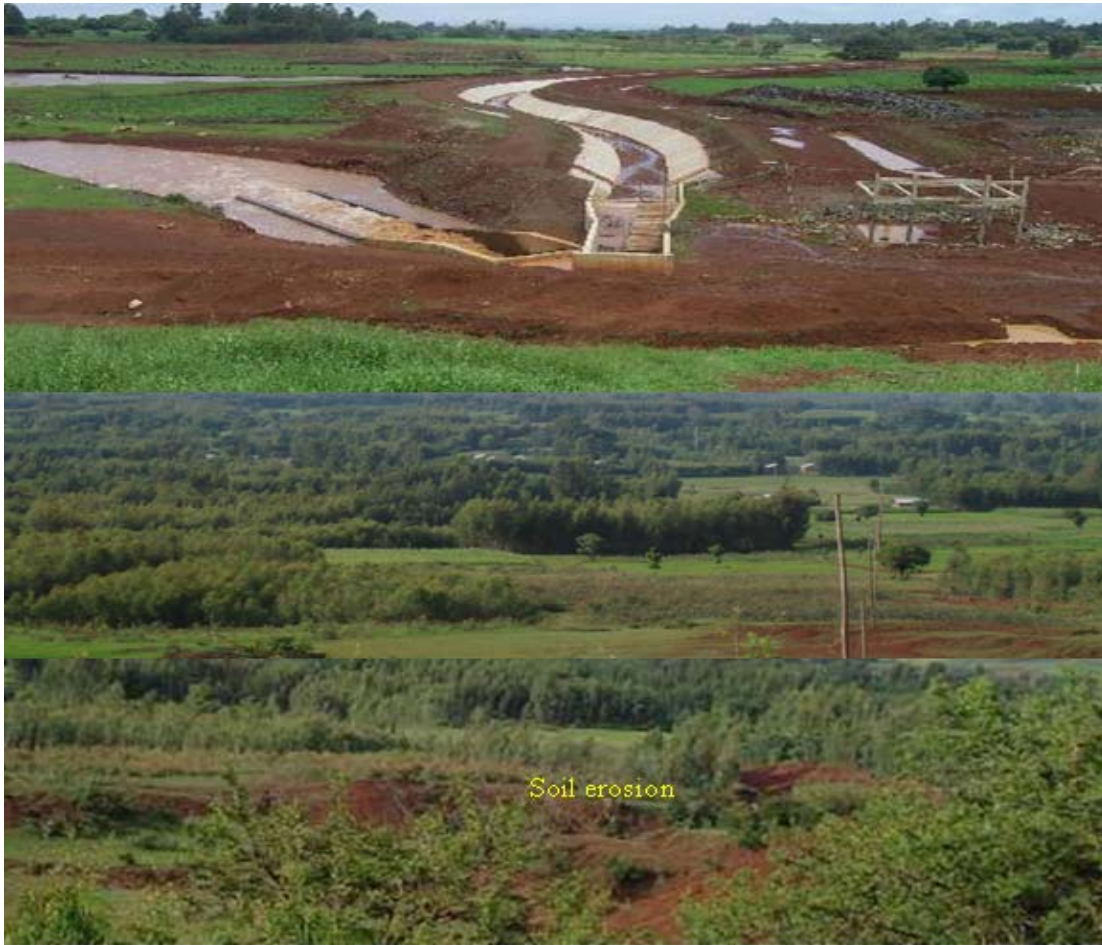
Figure 1: The Irrigation scheme in partial view of the Koga Watershed (Photo, in August 2008)
